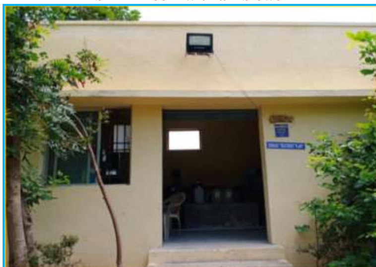
STP – Room with air blower
